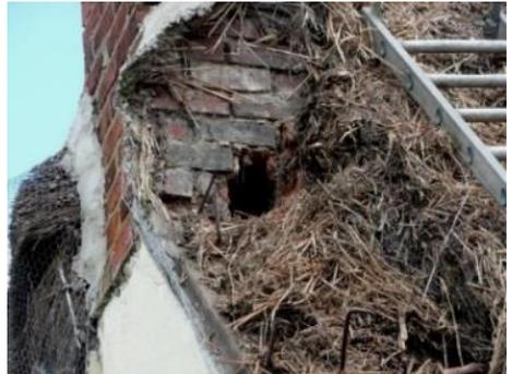
A spark arrestor can become blocked with tar deposits, which in turn can slow down flue gases leaving the chimney and build up heat in the flue. The general consensus is that if you don't have a spark arrestor, don't fit one.
